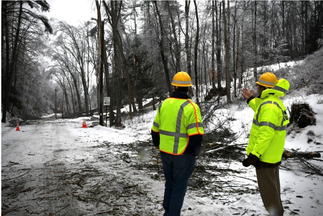
Central Hudson President and CEO Charles A. Freni and Vice President of Electric Engineering and Operations Ryan Hawthorne survey damage in Rosendale on Monday.
